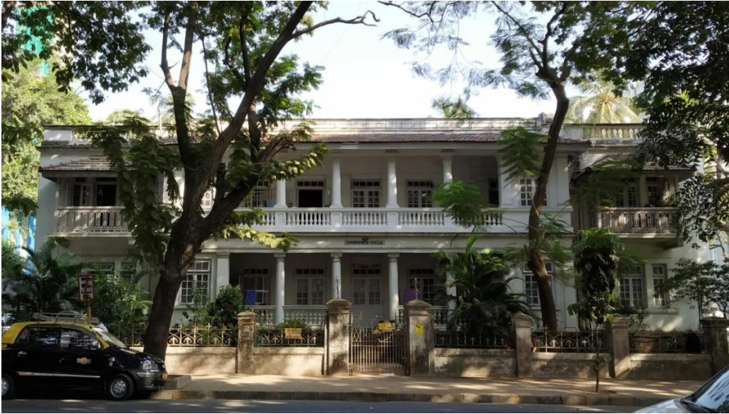
Photo above: Khursheed Villa, one of the oldest buildings in Dadar Parsi Colony-Photo by: Hormuz Bana
